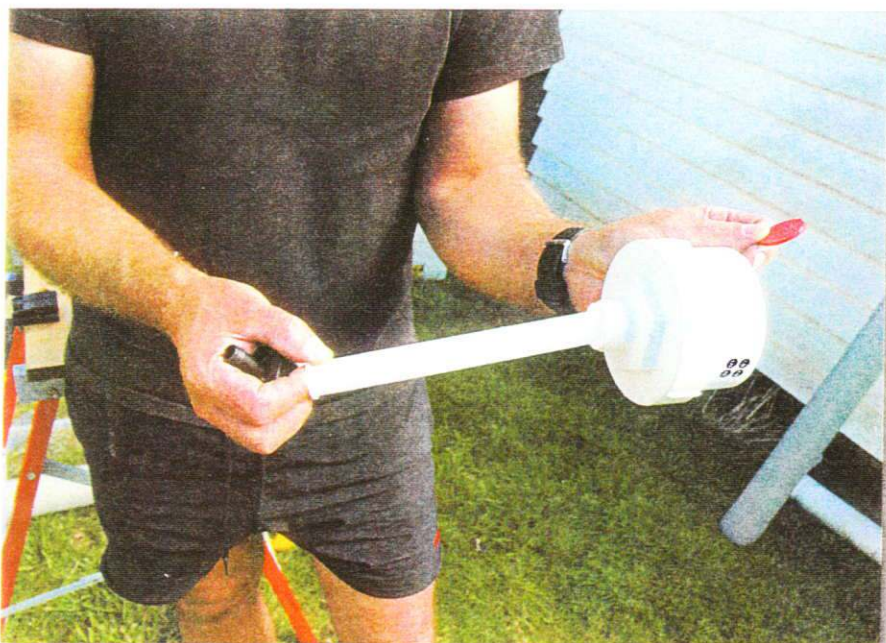
Plastic filter inside first flush diverter.
